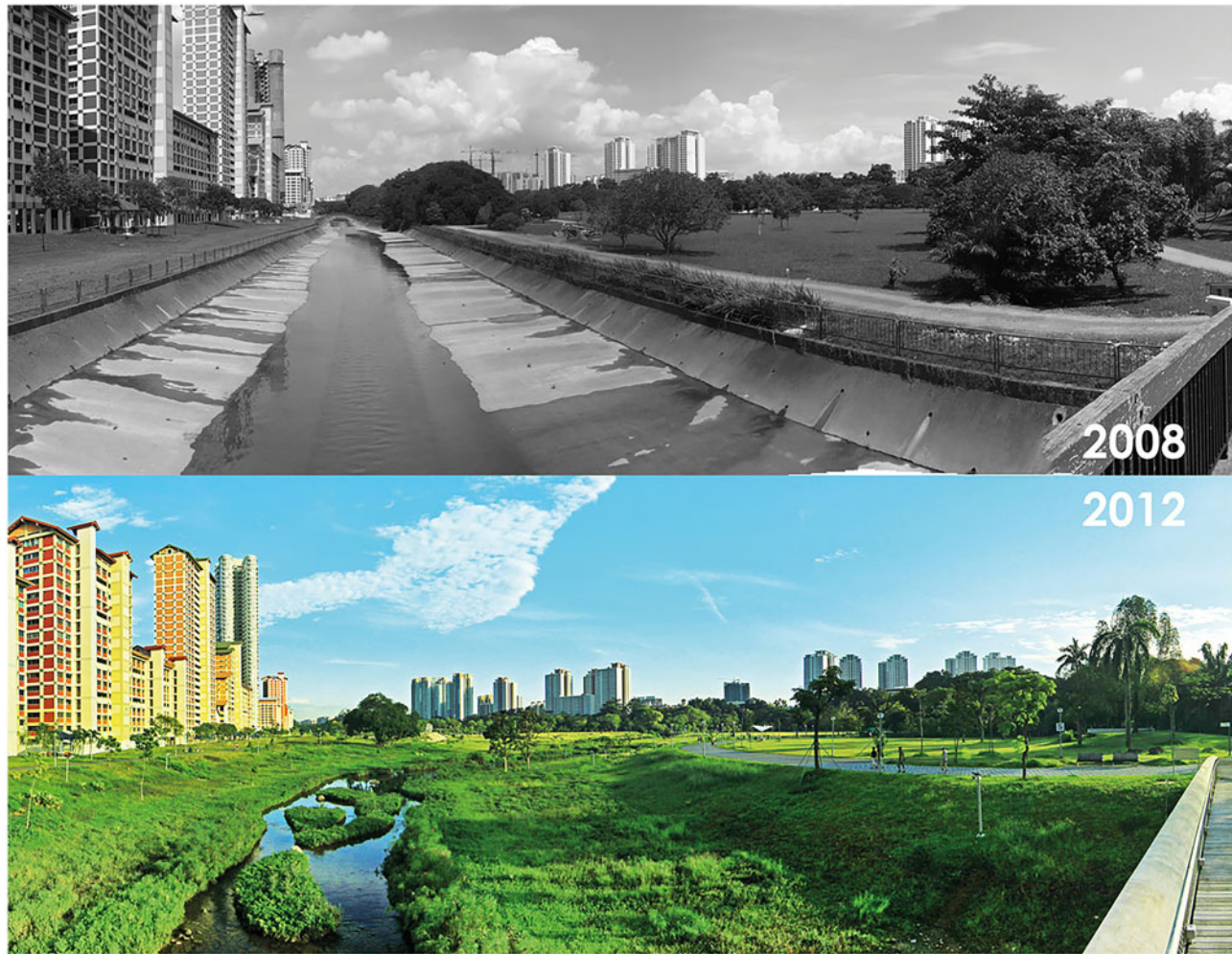
Figure 4: Bishan-AMK Park before and after the BGI interventions. Source: ASLA (American Society of Landscape Architects Professional Awards 2016a,b)
