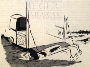
1954 THE HAZARDS OF THE SAND ROAD
